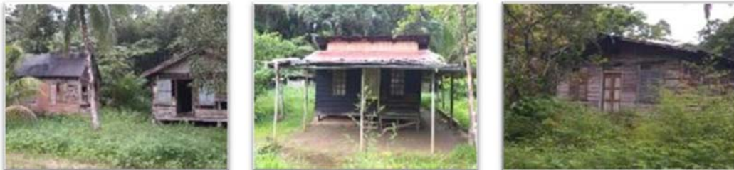
Photo 19: Abandoned houses at Hanover plantation (Source: Social Solutions, 2019)
