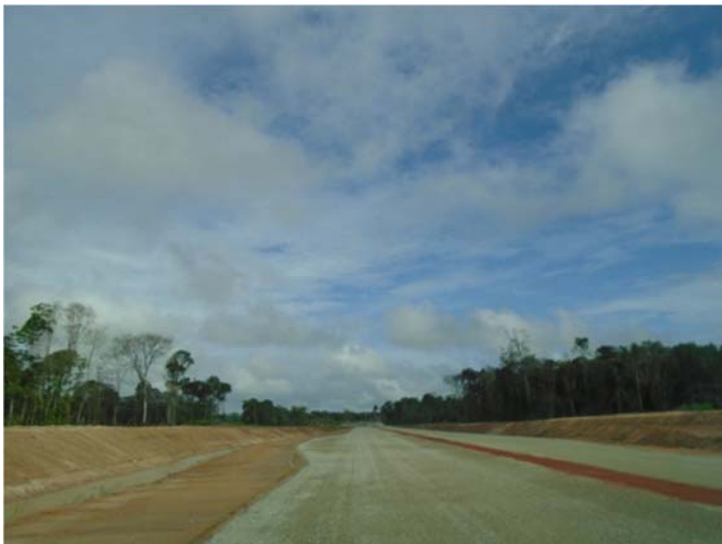
Photo 1: The Afobakaweg-JFK Highway connection road under construction
