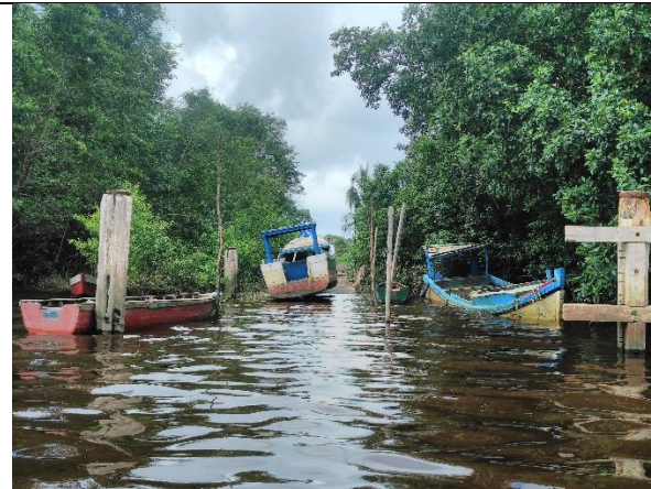
Old jetty, still used by some fisher boats. Cable will be placed on the left side.
