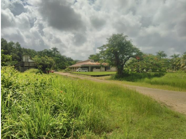
RGD Health centre, on east side at the end the Bamistraat
